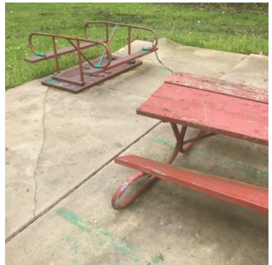
Picnic tables need to be repaired and/or replaced.
